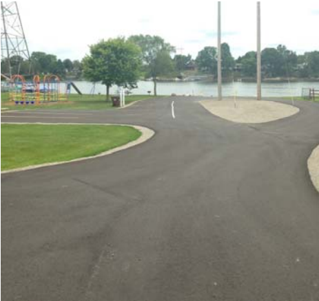
Somerset Park Parking Lot & Playground Equipment
