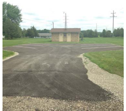
New Parking Lot & Driveway at Southern Shores Park
