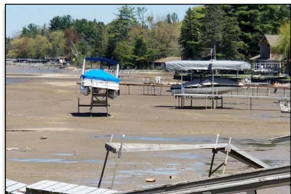
Sanford Lake - after 2020 dam failure
