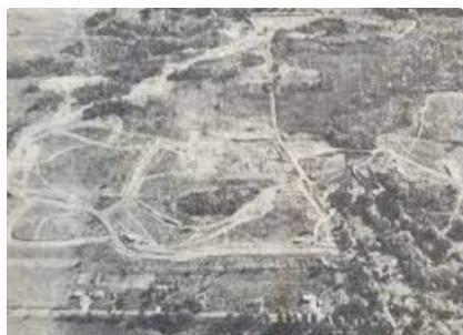
Clearing the Land
